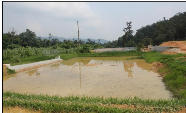
Plate 5.12: Example of Sediment Trap
