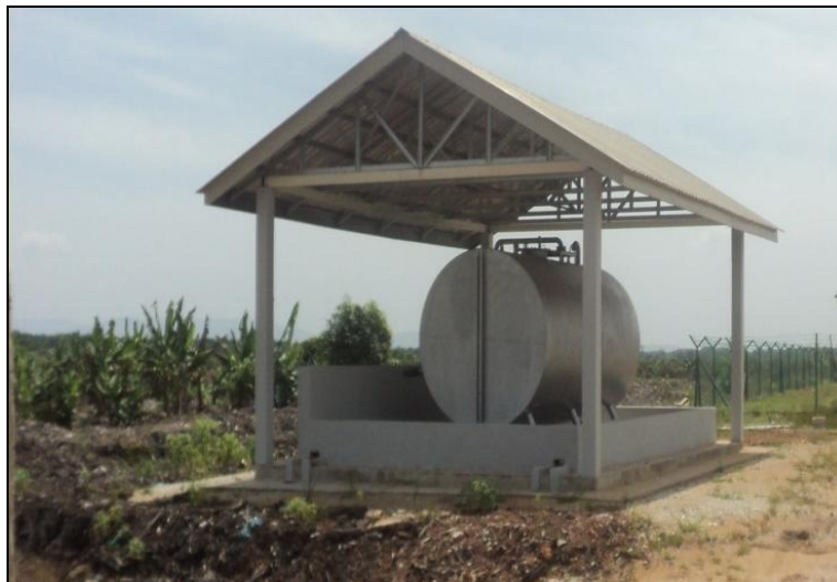
Figure 5.7: Example of proper storage skid tank with bund wall
