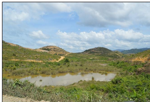
Plate 5.11: Example of Sediment basin at valley area
