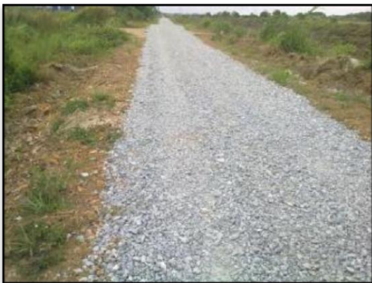
Plate 5.6: Example of Stabilized Access Road with Crusher Run
