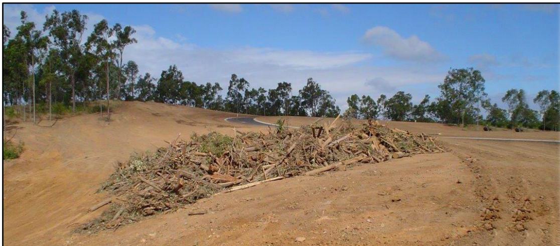
Plate 5.4: Mulching BMPs application locally in a land development project
